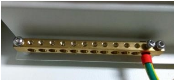
Figure 3.9 Grounding terminal block on the metal bracket
