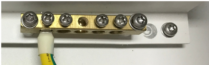
Figure 3.9 Grounding terminal block on the metal bracket
